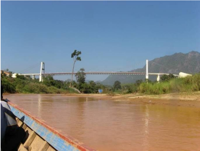
The 1000 feet long Leili bridge seen from the Pinlaung river towards north.
