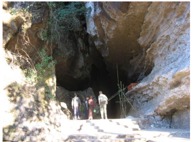
Entrance with construction of side platforms
